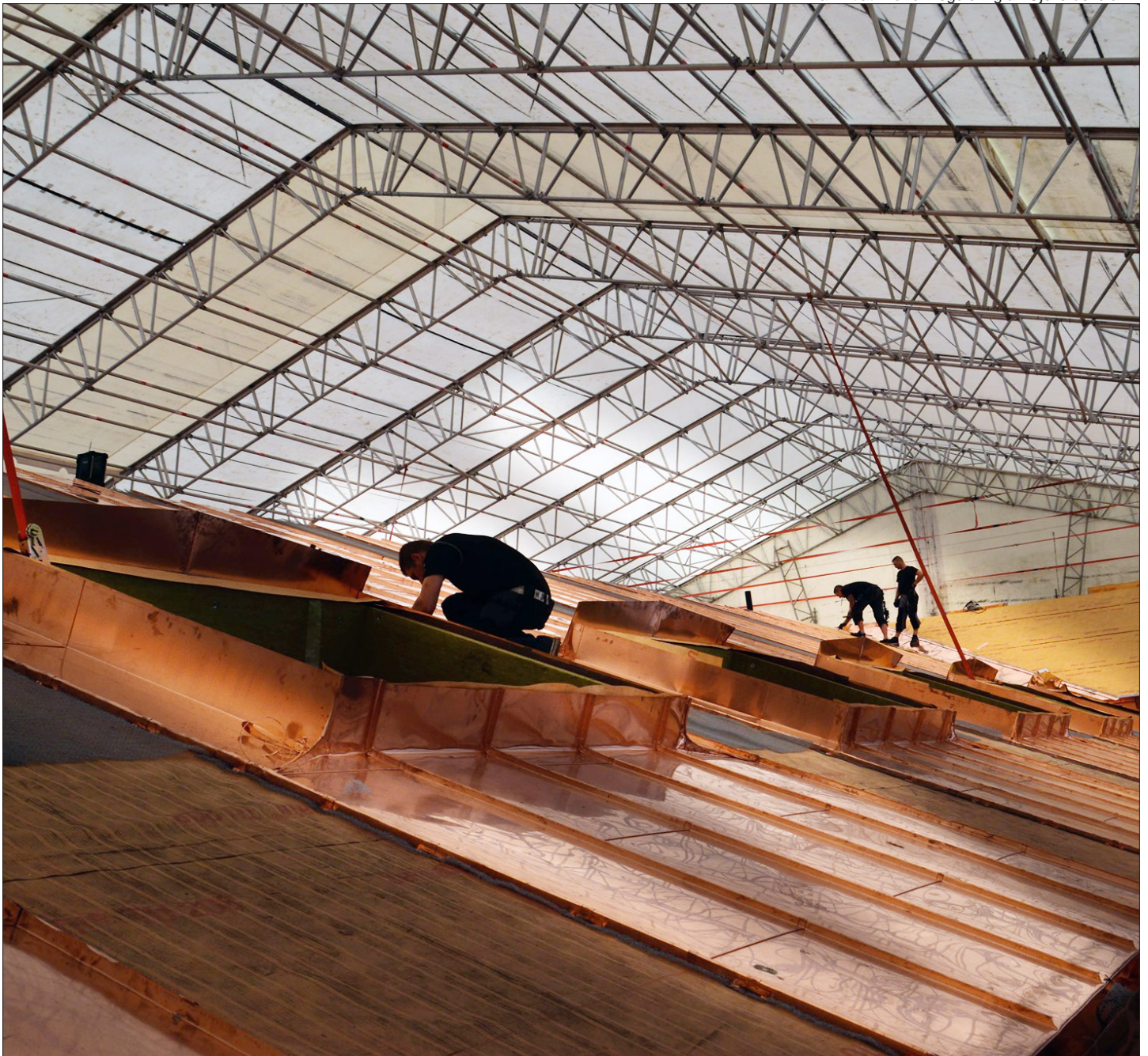
Karlsen & Nordseth AS i arbeid.
